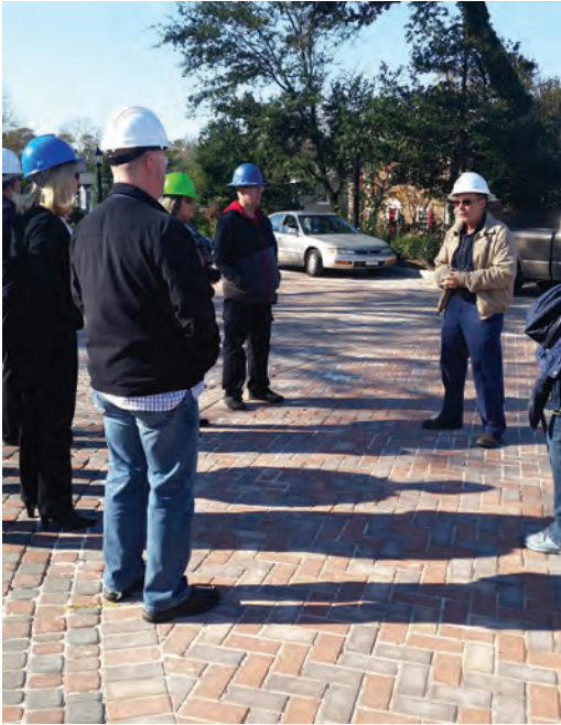
Entering the Cavalier construction area – a good view of the environmentally-friendly pavers being used throughout the property.
