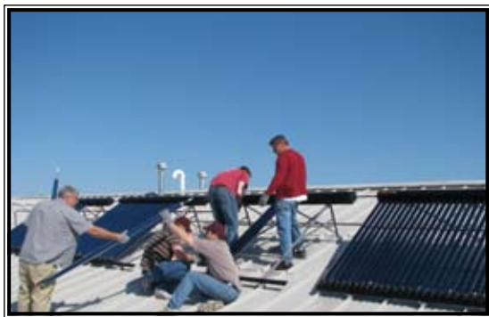
Larry LaRue (standing) inserts solar tube into collector
